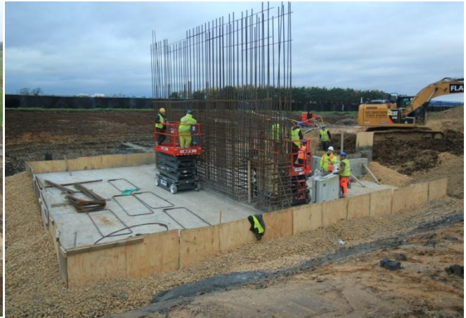
Fixing steelwork to central dividing wall
